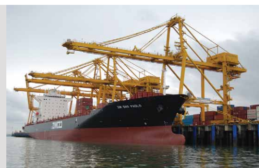
INCHEON CONTAINER TERMINAL
